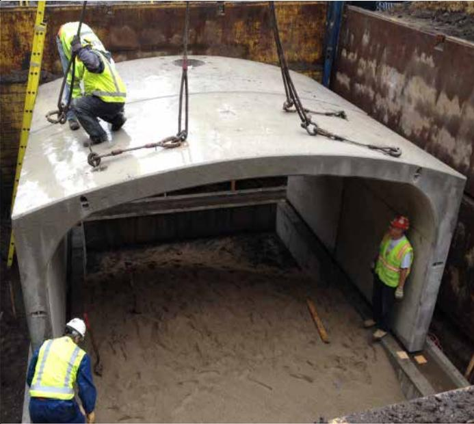
*The Back Cove Combined Sewer Overflow (CSO) conduit will create a storage system for sewer and stormwater runoff during rain events. This and other types of projects will reduce pollution discharges to local water bodies. (Photo courtesy of Contech® Engineered Solutions.)*
